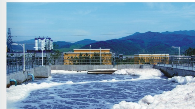
Sewage treatment purification
